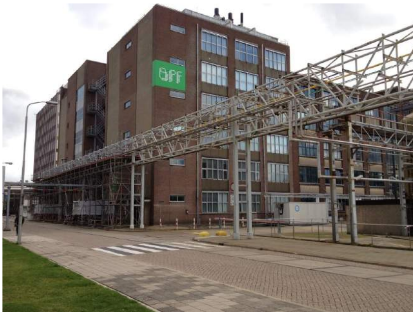
The Bioprocess Pilot Facility (BPF) in Delft
