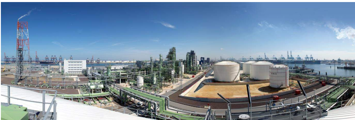
Neste Oil's renewable diesel (HVO) production plant in Rotterdam. (Copyright Neste Oil)
