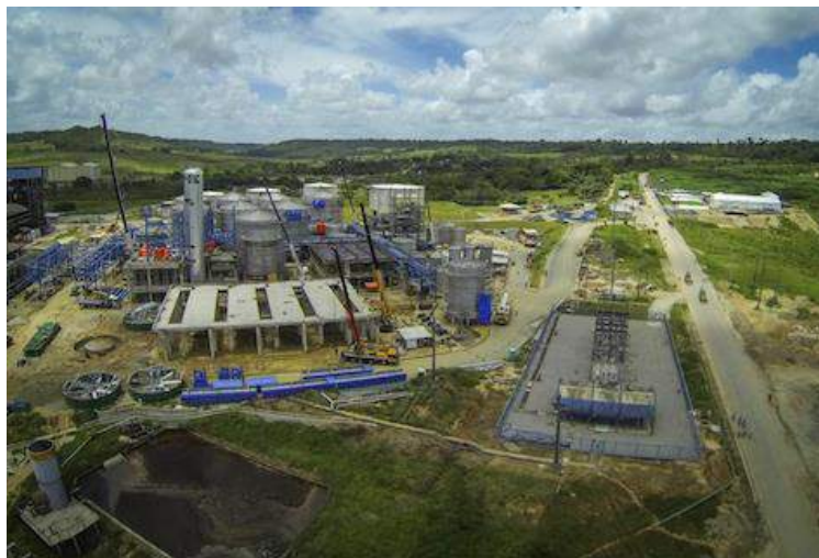
GranBio commercial cellulosic ethanol plant, Alagoas, Brazil.
