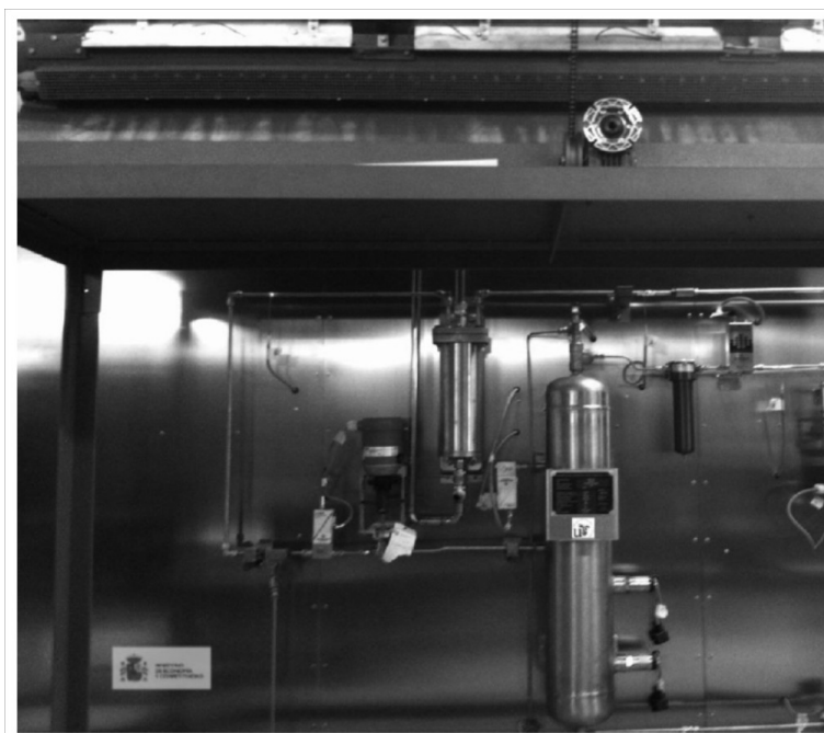
Fig. 2. General picture of the pilot plant
